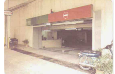
Floodgate Fully Open: (7'6" x 20'0")
